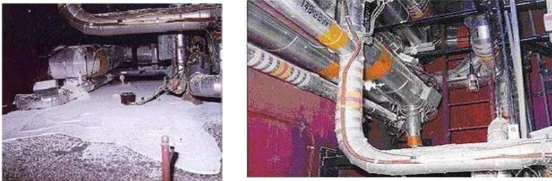
FIG. 6. Leaked Sodium on the Floor and Pipelines
